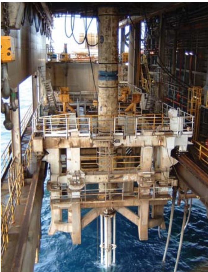
ROC's first deepwater well, offshore Equatorial Guinea
